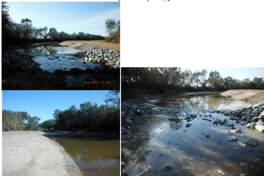
Coffer Dam at removal and waters flowing into the newly excavated Salt River Channel 10/09/2013.
